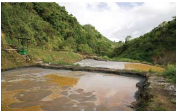
Coopellanobonito's water-cleaning facilities, Llano Bonito, Costa Rica, ©2009, Eduardo Martino
